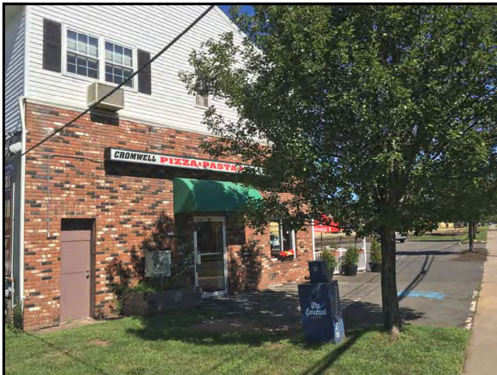
VIEW OF EAST SIDE OF SUBJECT BUILDING
