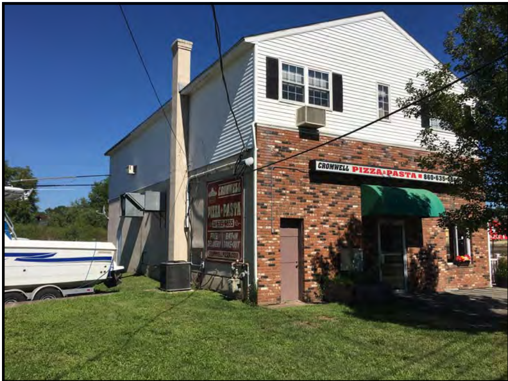
VIEW OF SOUTH SIDE OF SUBJECT BUILDING
