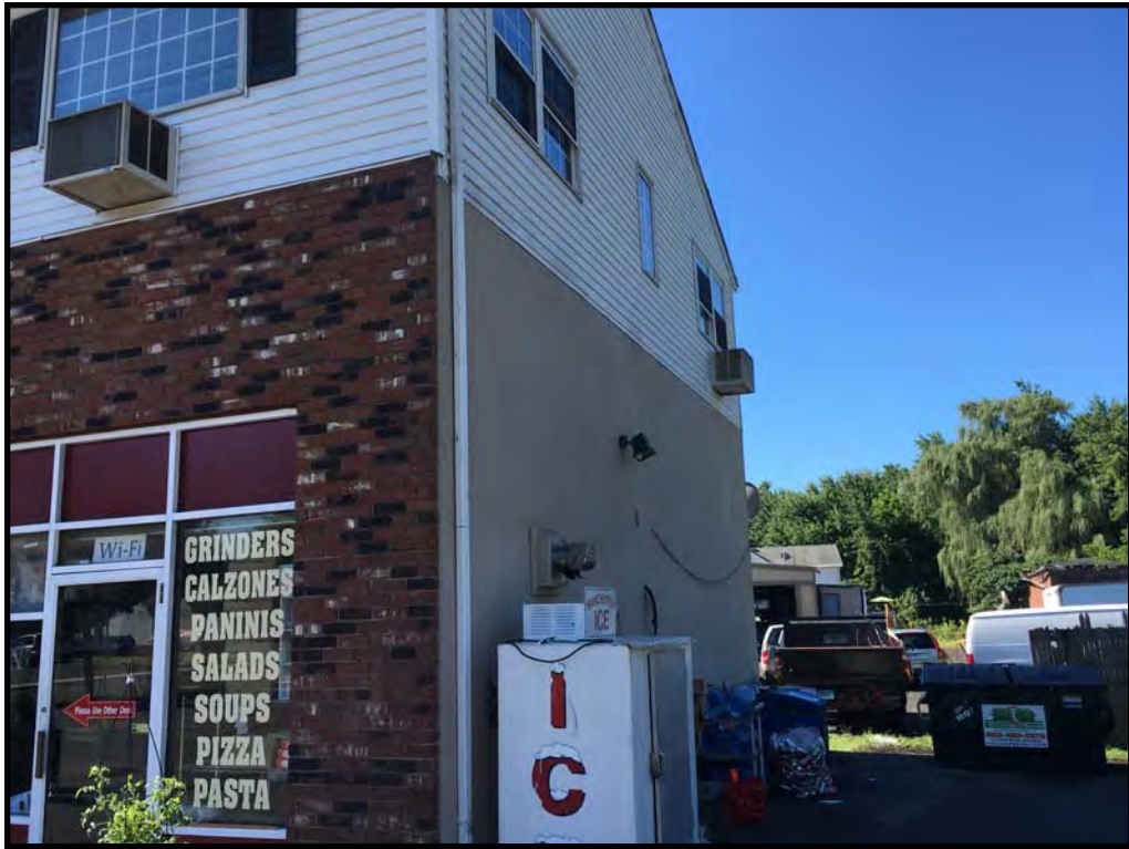
VIEW OF WEST SIDE OF SUBJECT BUILDING
